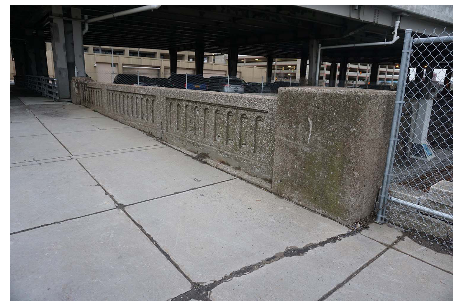
View of CSX Bridge Guardrail
