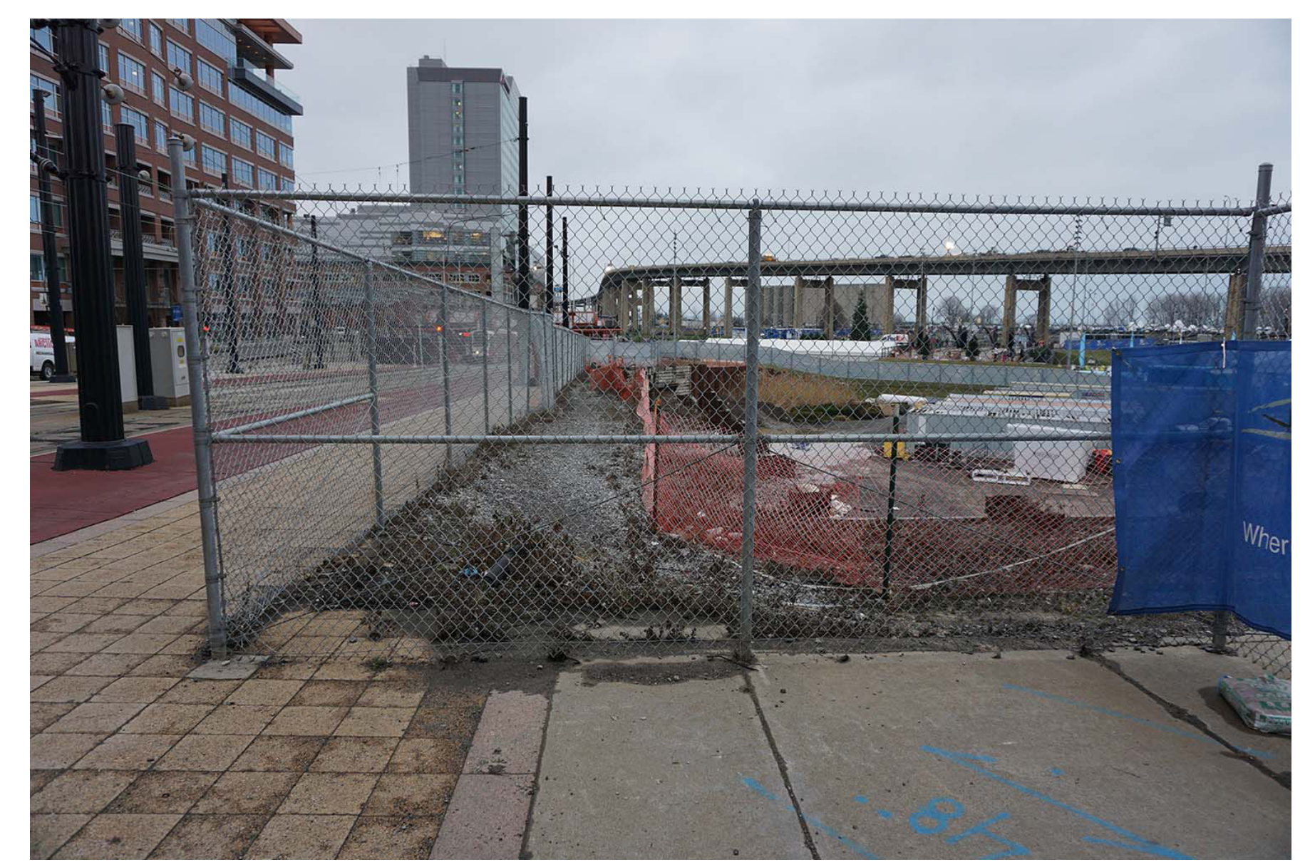
View South to Existing Aud Block
