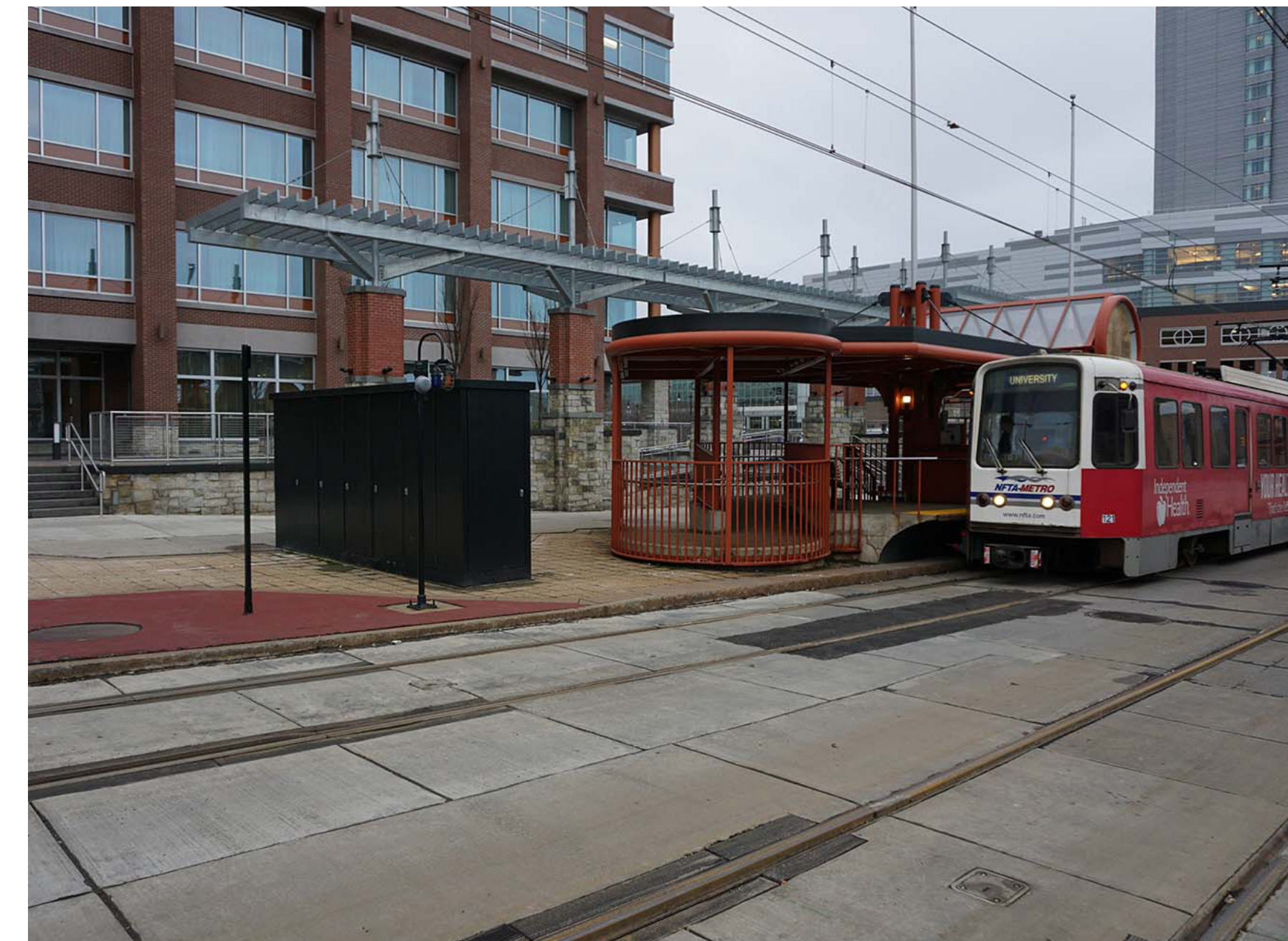
View East to Northbound Metro Rail Station and One Canalside
